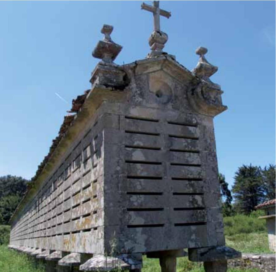
The original and seemingly mysterious buildings with a cross on the roof, which you can see while going through Galicia, are the so called horreo - granaries raised from the ground by pillars for protection against pests.
